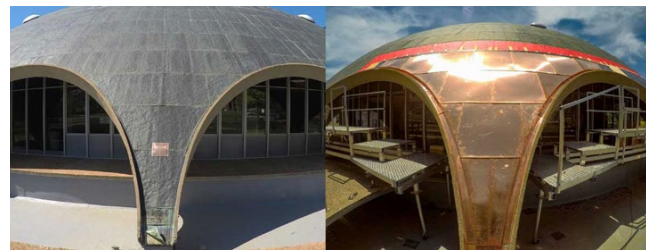
The Shine Dome is being restored, beginning with the curves of the arches. Photos: Australian Academy of Science
