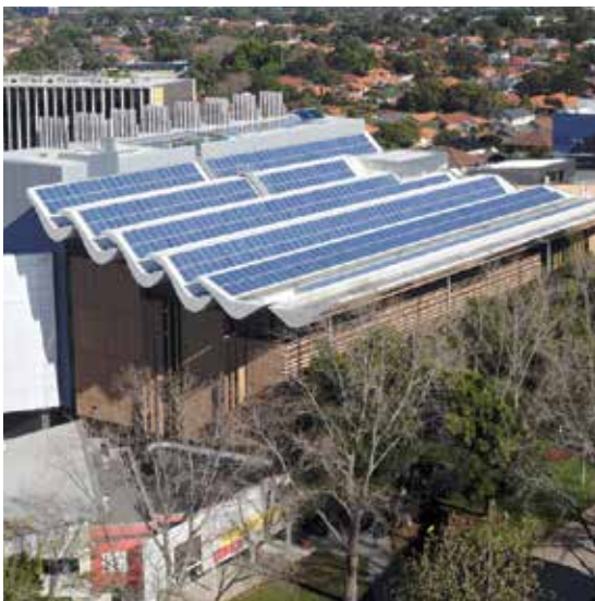
Figure 12: The ‘Six Green Star’ rated Tyree Building, UNSW. Image courtesy SPREE, UNSW
