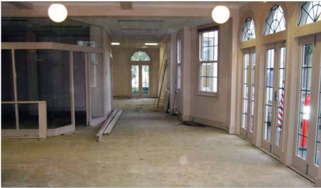
Ian Potter House during the refurbishment process
