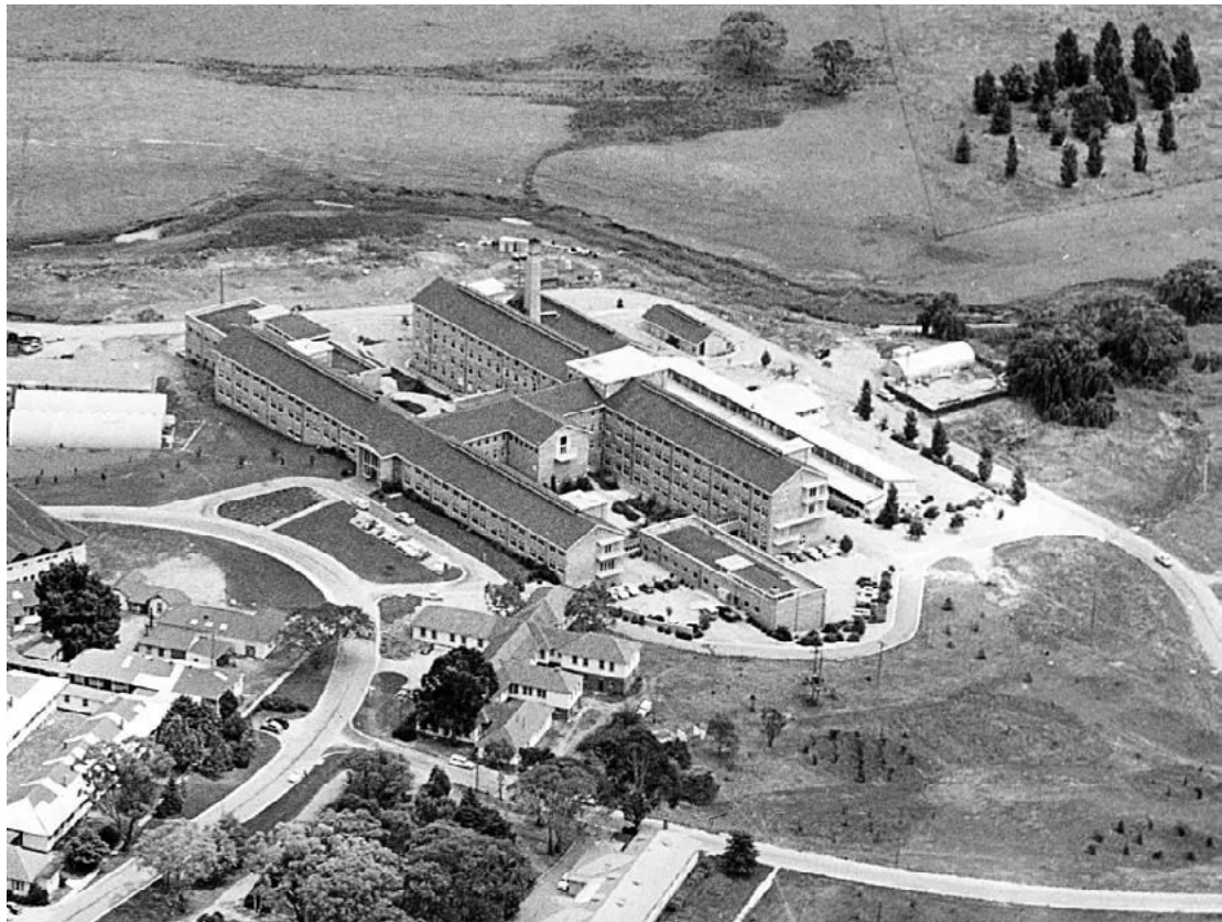
Fig. A57. The original ANU Research Institute's buildings in Canberra A.C.T. [CA]
