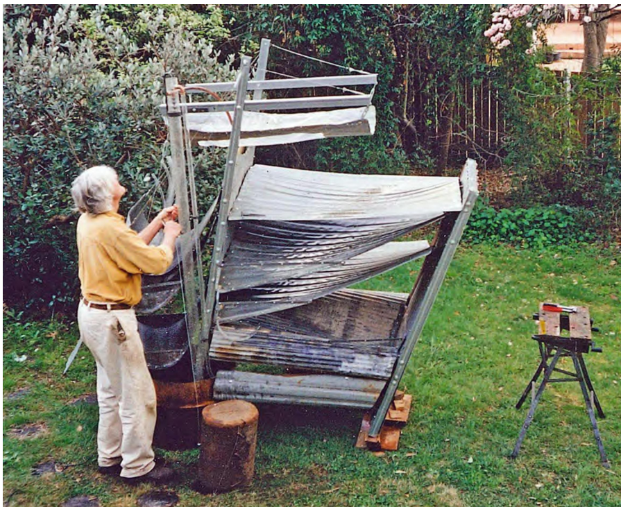
Fig. 9. Waterstress installation under construction by John Chappell.
